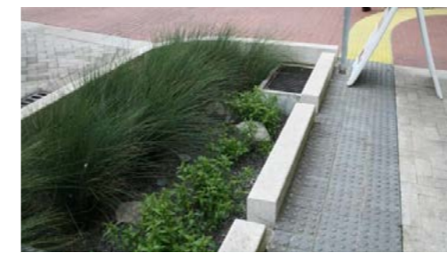
Rain gardens collect, slow and clean runoff.
