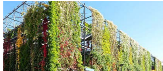
A natural multi- Storey car park facility
