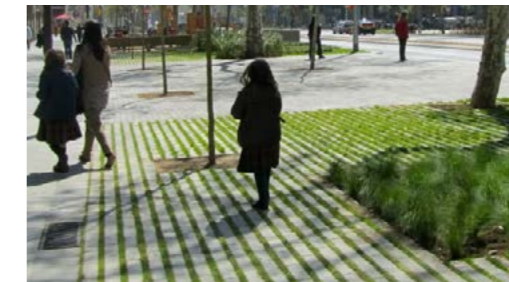
Incorporating permeable surfaces into streets will assist in flood mitigation by allowing water to infiltrate the ground.
